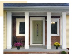
the columns aren't susceptible to damage or movement if the underlying post twists (as pressure-treated posts have been known to do). And the built-in wiggle room allows the columns to be lined up perfectly along the front of a porch or deck even when the structural posts are a little off.
