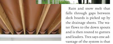
it protects deck framing from water damage, something below-joist systems do not. It's also easy to install, requiring only a utility knife, a staple gun, and a caulk gun.
